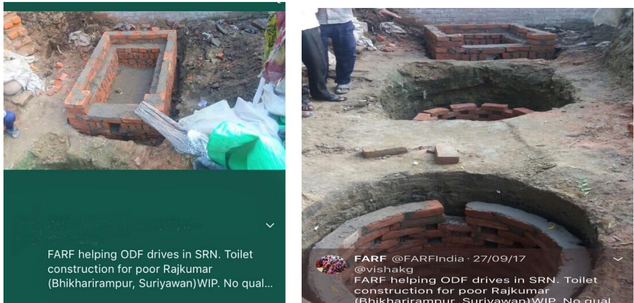
Picture 3: Initiatives taken by FARF for construction of toilets
